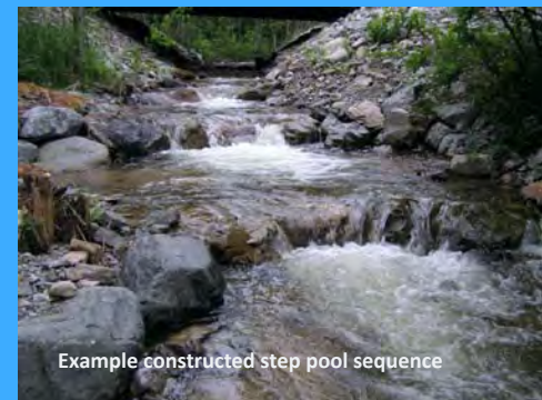
Example constructed step pool sequence
