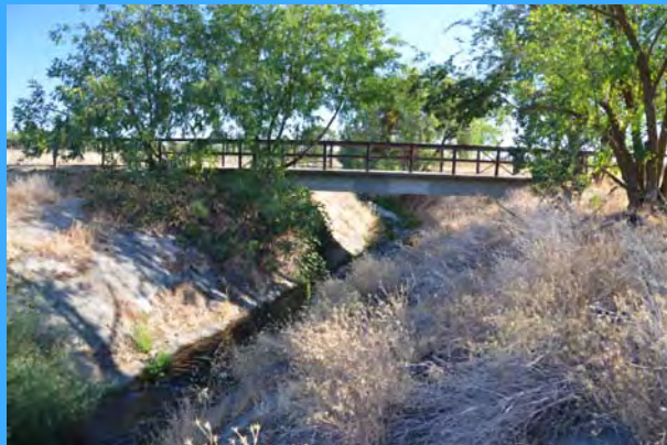
Parkway bridge to remain
