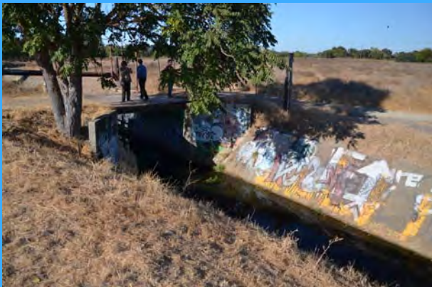
Existing bridge to be removed
