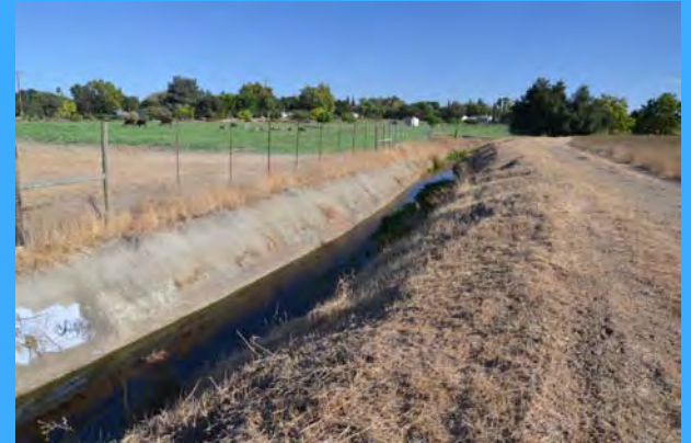
Existing concrete lined trapezoidal channel
