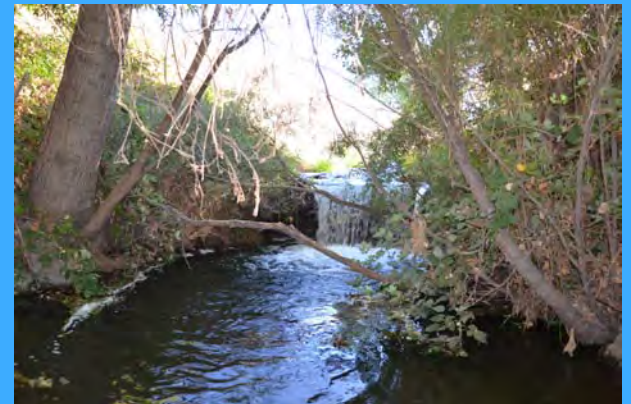
Failing concrete channel at outfall (or "headcut")
